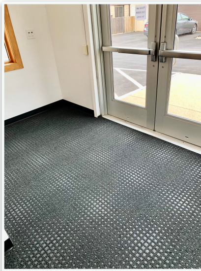
New carpet squares installed in stair landings.
